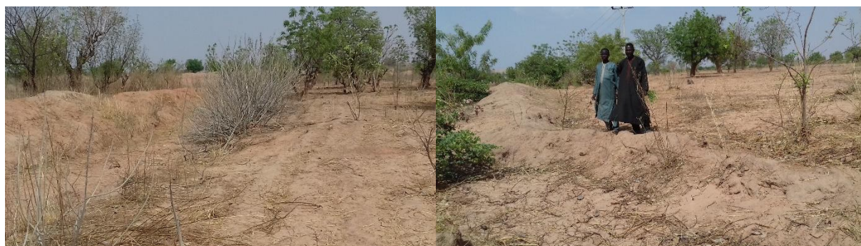
Earth embankment and shrub planting for water erosion control in Laye VA (Yobe State).
