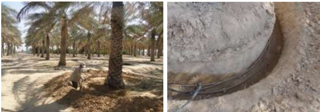
Figure 6. Preparing the subsurface water distribution system at a depth of 50cm
