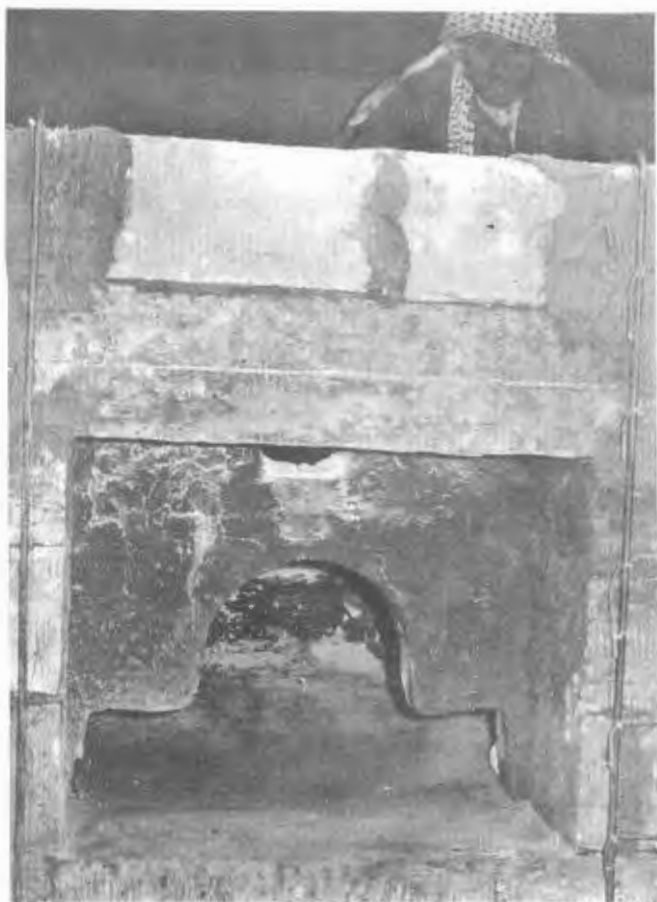
Fig. 2. The doorway of the khobz oven.
