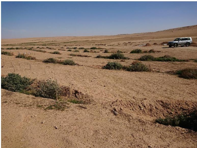
Figure 6 Vallerani structures in the treated sub-watershed
