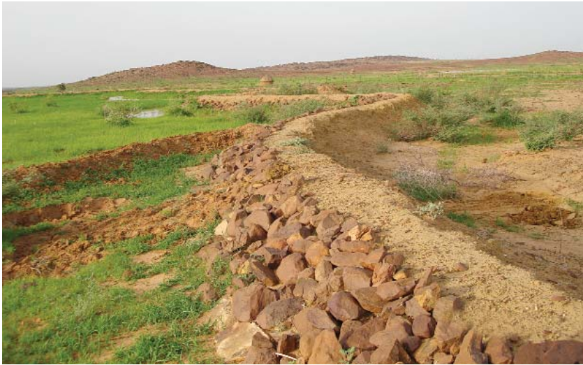
Low-cost contour ridges have proved remarkably effective in fighting erosion and improving soil moisture in several countries in North Africa.
