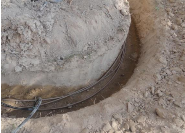
Fig. 2. Installation of the subsurface drip lines around tree
