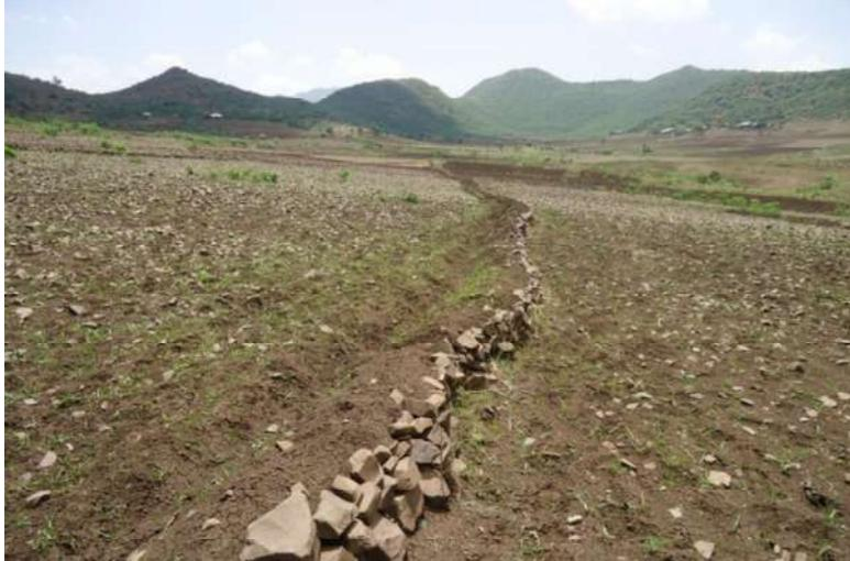
*Figure 2. A stone bund located in the treated sub-catchment (Ayaye) of Gumara-Maksegnit watershed.*
