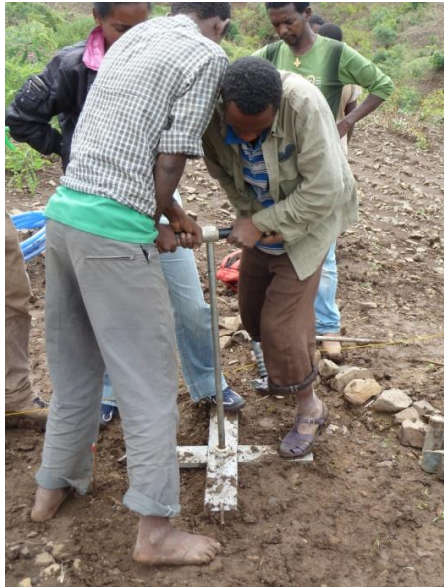
Drilling the hole
