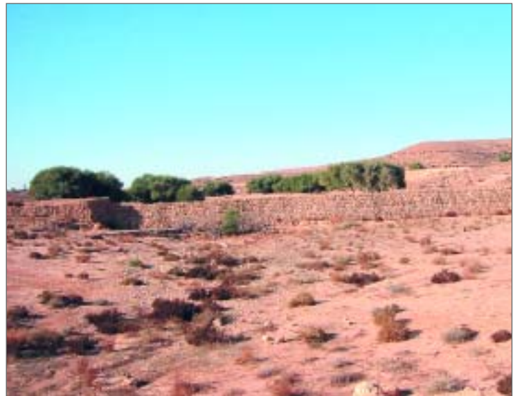
Jessour water-harvesting system in Oum Zessar watershed, Tunisia: olive trees prosper on the runoff water and sediments captured by the stone dike.
