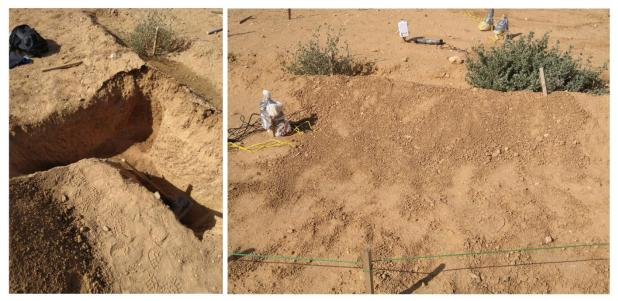
Figure 10 Left: Picture of the cut used to install the Decagon 5TE sensors. Right: The Vallerani RWH structure after the cut was filled up.
