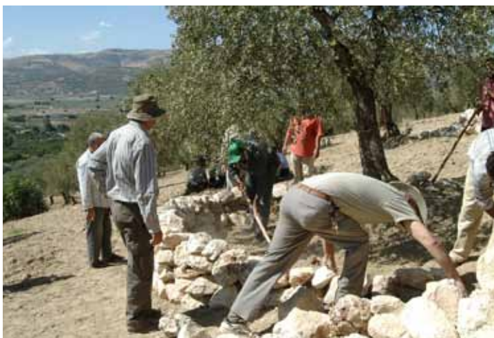
Science plus self-help: the community in Afrin builds simple stone structures to reduce water runoff and soil erosion.
