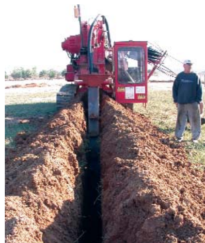
Installation of subsurface drainage pipe using specialized equipment.
