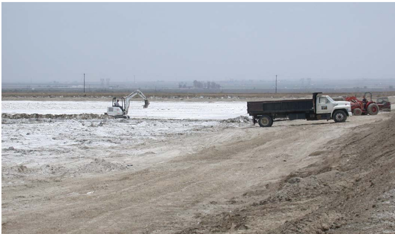
Accumulated salt is removed from an evaporation pond, one option to manage salt on-farm.
