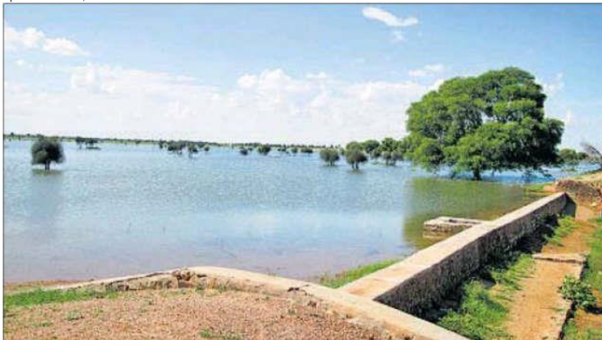
Rainwater being harvested in (masonry) check dams in Govindpura.
