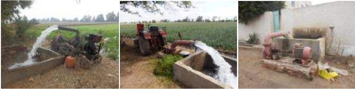
Well with suction pump
