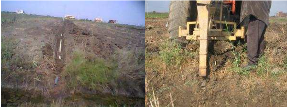
Drain installation
