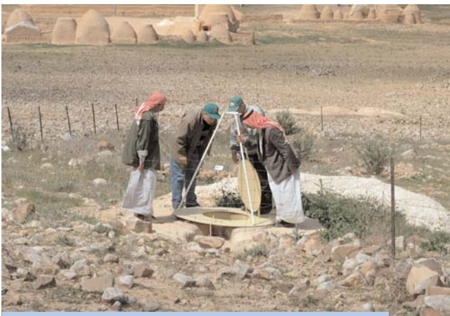
Indigenous Roman-type cisterns are being used in Khanasser village to collect runoff water to irrigate olive trees during summer.
