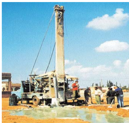
Drilling a well in the study area
