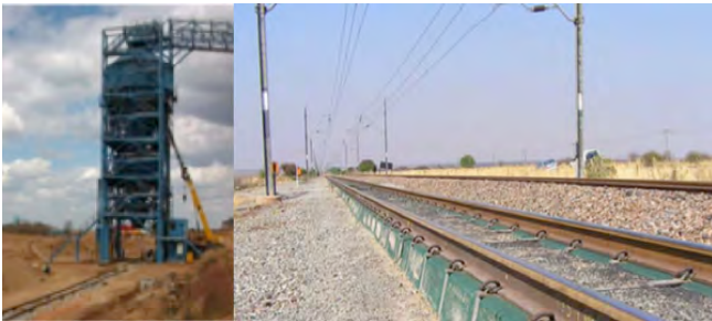
FIGURE 2. FACILITY FOR COAL LOADING IN TETE PROVINCE AND IMPROVED RAILWAY LINE TO FACILITATE IMPORT-EXPORT.
