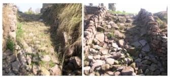
Figure A5 Front view of conservation structure built using local available stones
