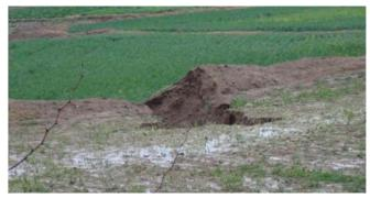
Figure A2 Breached terrace bund/embankment
