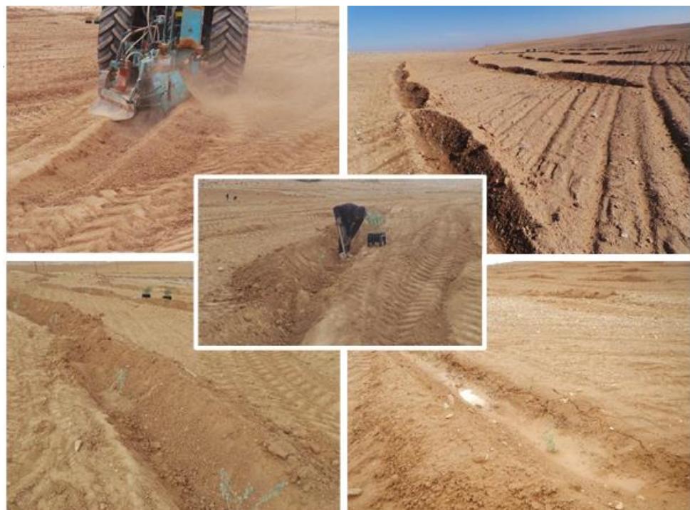
Figure 5. Intermittent contour ridges for capturing excess rainwater runoff on slopes
