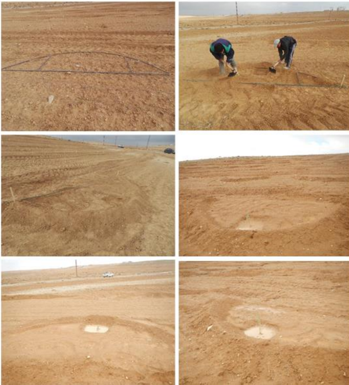
Figure 6. Preparation of semi-circular bunds for forage shrubs
