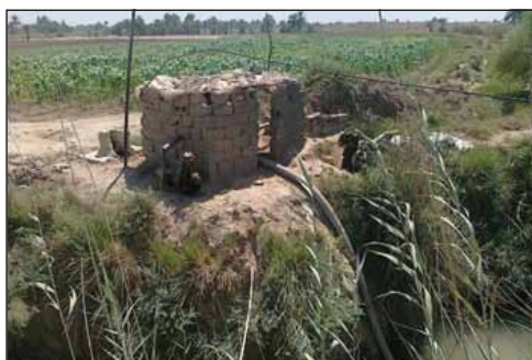
Figure 25. Irrigation pump installed by a farmer on an irrigation canal to combat low water levels in the canal.
