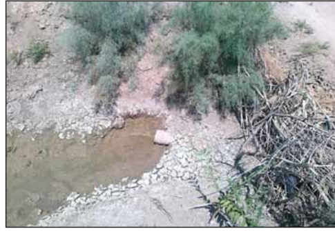
Figure 28. Illegal water-off take from a main canal.
