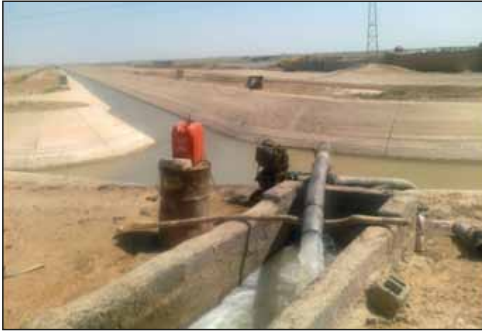
Figure 27. Unapproved pumping of water from a main canal.
