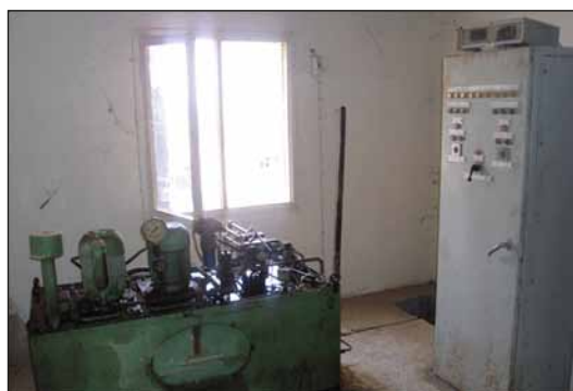
Figure 23. Remains of a control system for a main regulator at the Dujailah Irrigation Project.
