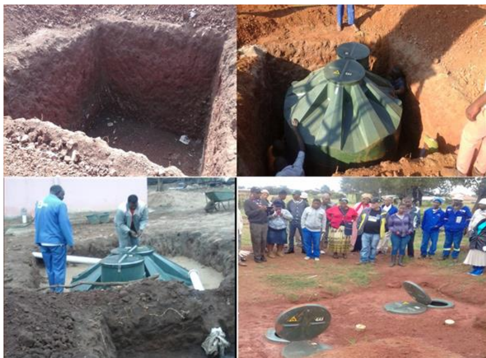
Figure 2. Biodigester installed at one of the sites in Free State, South Africa
