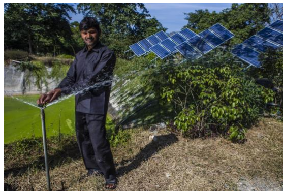
Figure 2. Sprinkler system energized through a submerged solar pump.
