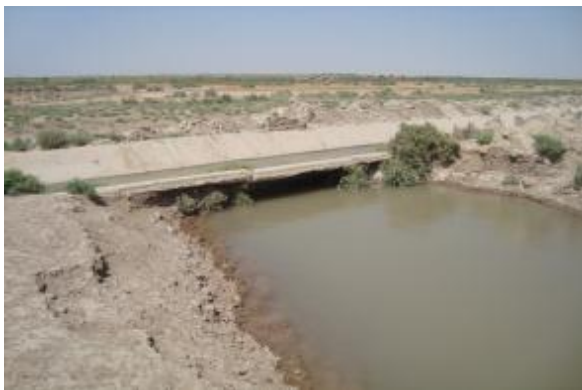
Figure 4: Damaged concrete lining.
