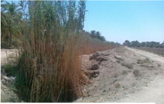
Figure 5: Wild growth in drainage channels at Mussaib
