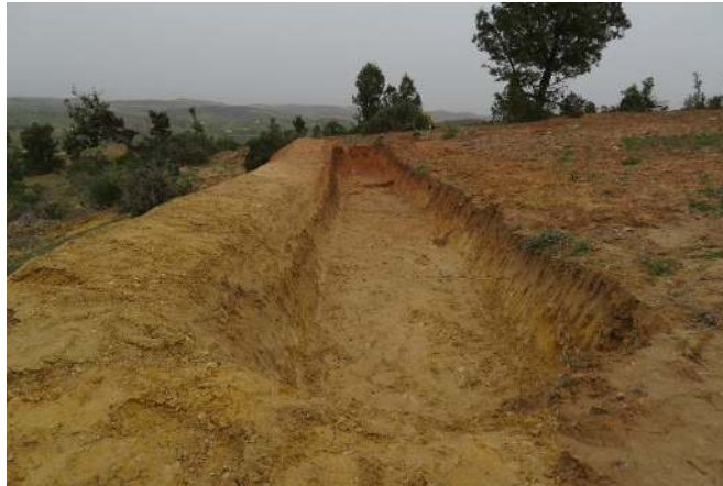
Figure 19. Benches constructed manually at Sbaihia pilot site, Tunisia (Winter 2018)
