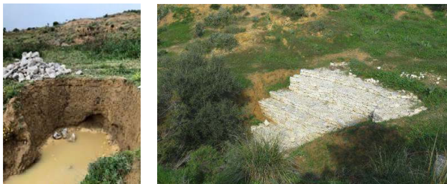
Figure 18. Stone gabions constructed within the Sbaihia pilot site, Tunisia (Winter 2019)
