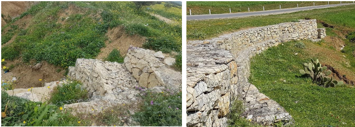
Figure 26: Stone threshold in Sbaihia, (Zaghuan) in order to stop down the gullies formation.
