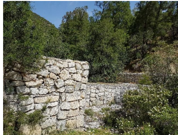
Figure 25: Gabion threshold in order to slow down the water flow in the wadi courses and improve its infiltration into the deeper soil in Sidi zid, (Zaghouan). Field photo, 23/03/2017.
