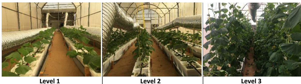
Figure 34- Cooled air flexible duct on three levels; the duct moves up with plant growth
