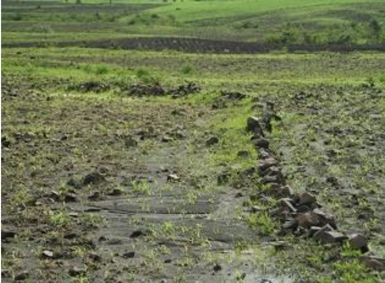
Figure 32: Stone bund; the area behind the bund did not fill entirely with sediments yet.
