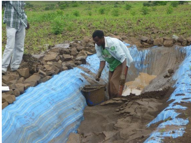
Figure 14: Removal of sediments using buckets
