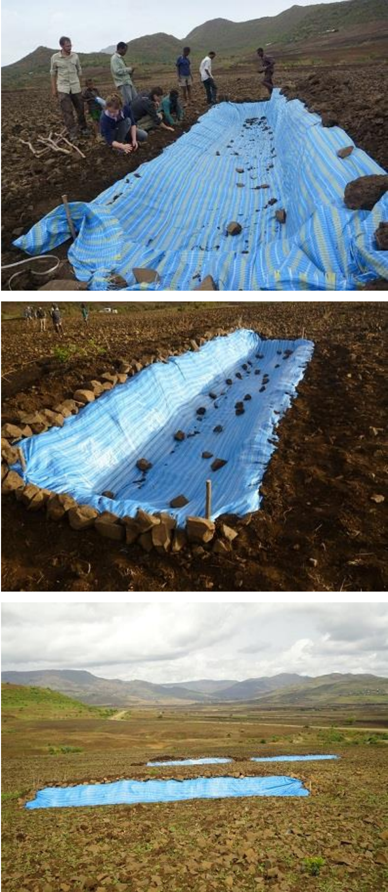
Figure 11: Construction of the sediment retention basins
