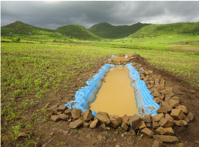
Figure 12: Sediment retention basins filled with water after rainfall events
