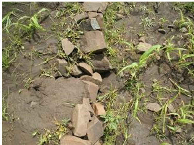
Figure 31: Sediments overtopping the stone bund
