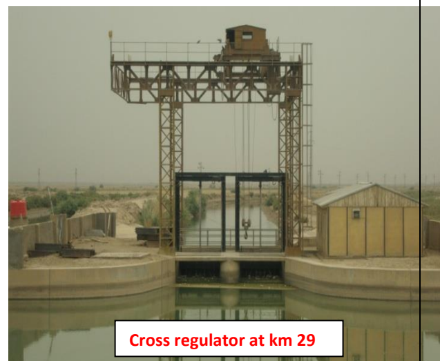
Figure 2: Irrigation network at the Al-Dujaila project area with a cross regulator at 29 km.
