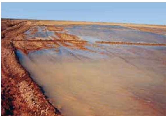
Fig. 2.2. Poor water distribution because of improper land leveling
