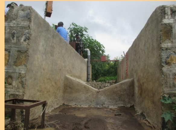
Automatic monitoring at the outlet of watershed and two sub-watersheds ( stone bunds- treated and untreated)
