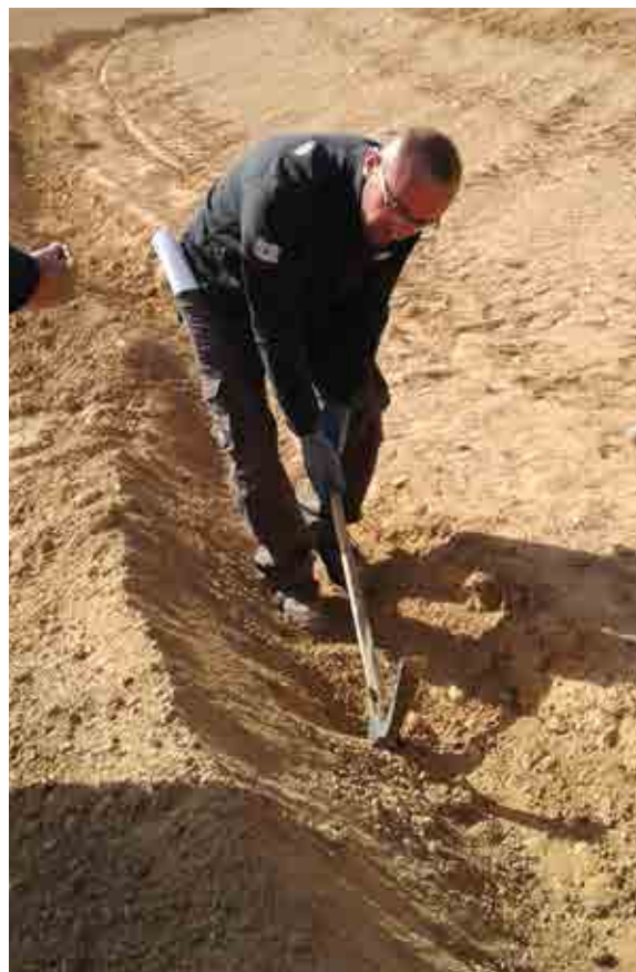
Digging a water harvesting pit in the Jordanian 'Badia.'
