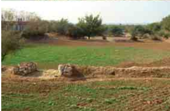
Runoff harvesting and soil-conservation structures installed in gullies
