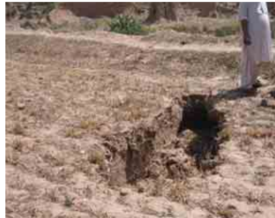
Figure 5.21. Soil hydraulic shear failure at the edge of a terrace
