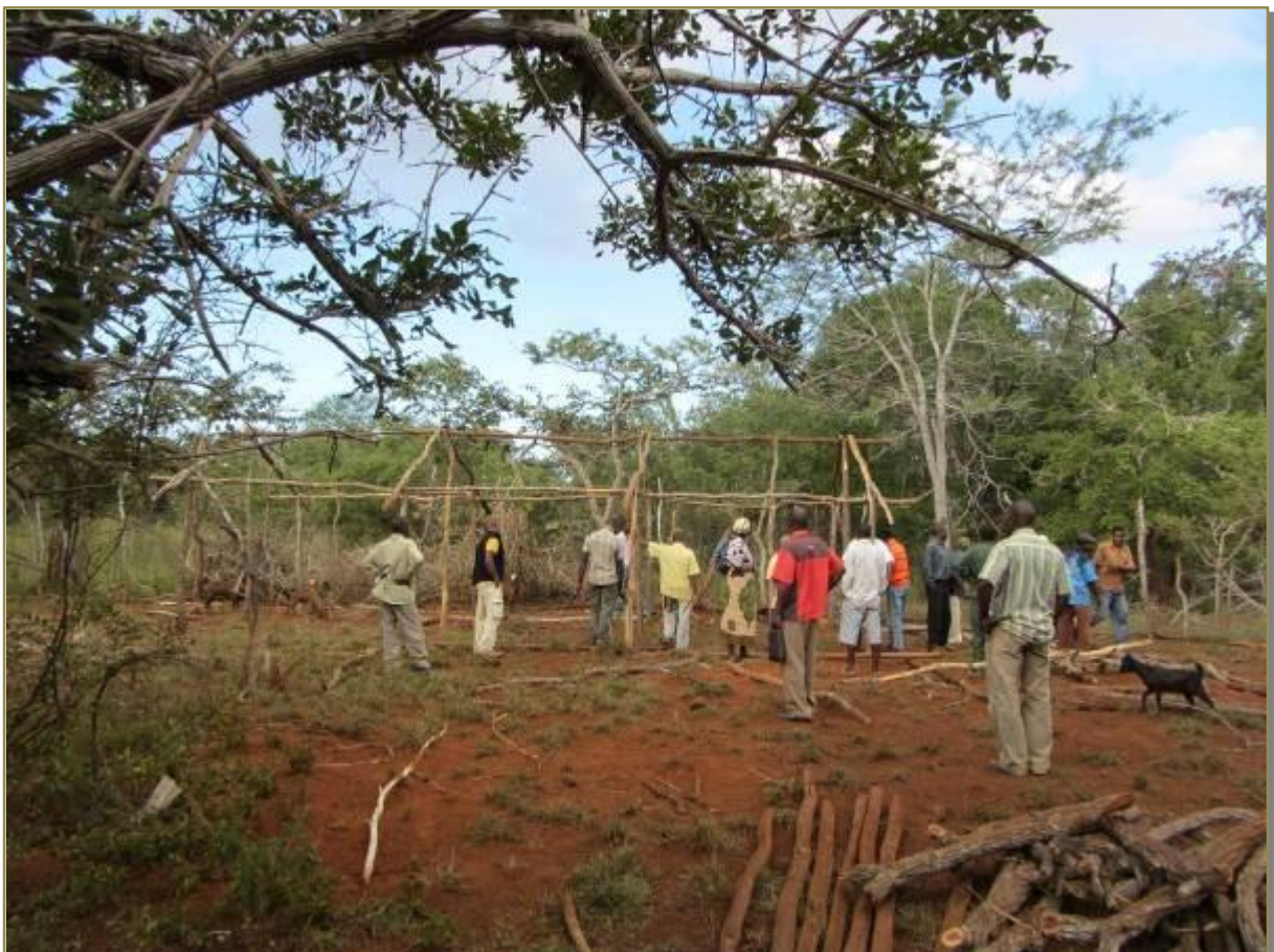
Figure 4. First steps of a (large) improved kraal in Vuca Interior.
