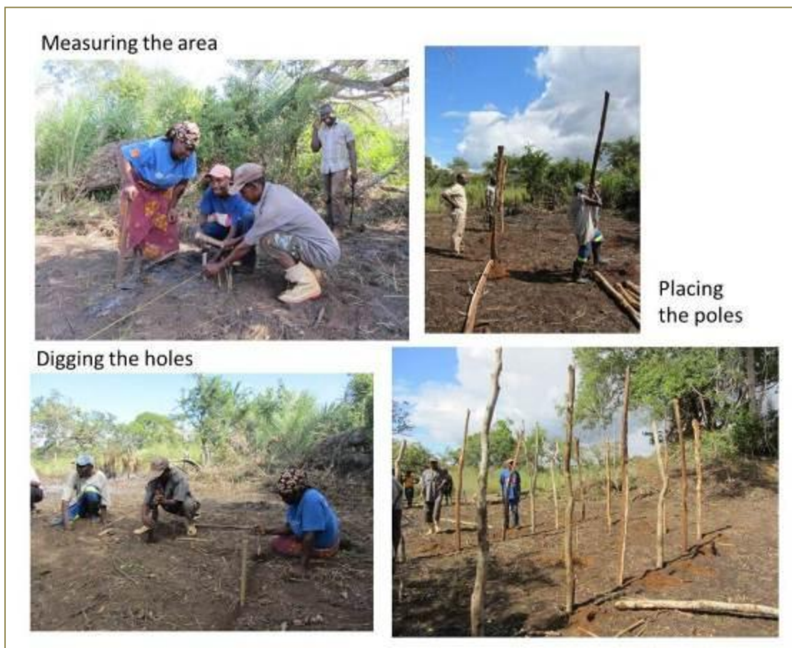
Figure 2. First steps in constructing the first improved kraal.
