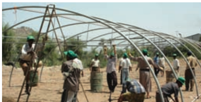
Low-cost greenhouse frames are made locally, and can be erected quickly
