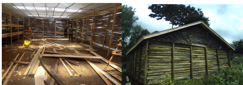
FIGURE 5. Potato Value chain. Left: Early stages of construction of diffused light store (DLS) for KWESTO FCS. Right: Completed outer structure of the DLS. The 50- tonne seed storage capacity DLS was constructed through cost sharing with AVCD- Potato component procuring the construction materials and Aphid proof insect net while KWESTO FCS provided labor for construction and a committee member provided land where the DLS has been constructed.
