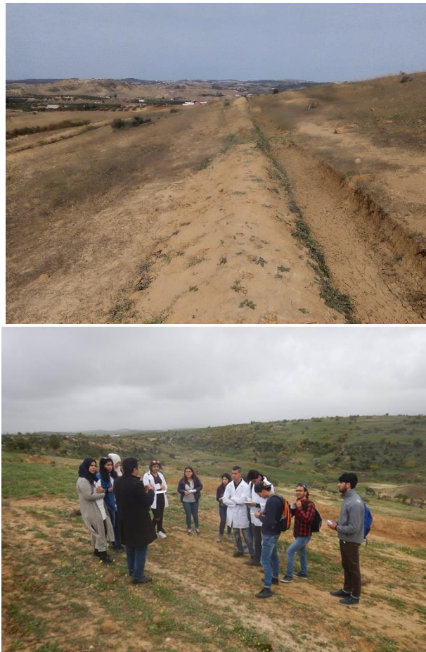
Figure 2. Benches constructed manually within the pilot site.
