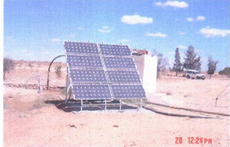
Figure 10. Wali, Menzel Habib/ Solar energy for pumping water at low pressure for irrigation of cash crops (Sep 2004).
