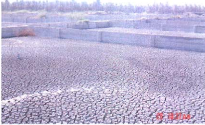
Figure 11. Drying in open basins of waste water sewage sludge
