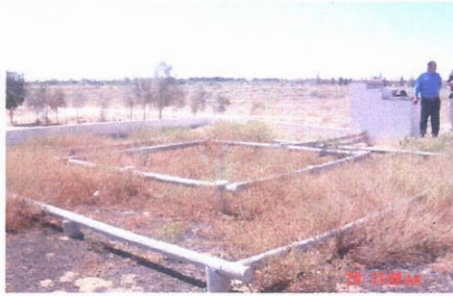
Figure 7. Dissa perimeter/filtration percolation station constructed by IRA Mednine (2002). Up ground view.
