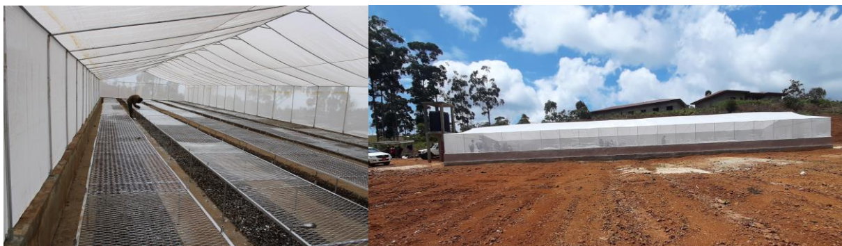
Figure 6. The inside view (left) and outside view (right) of the potato screenhouse built for IRAD in Bayangam, West region.
