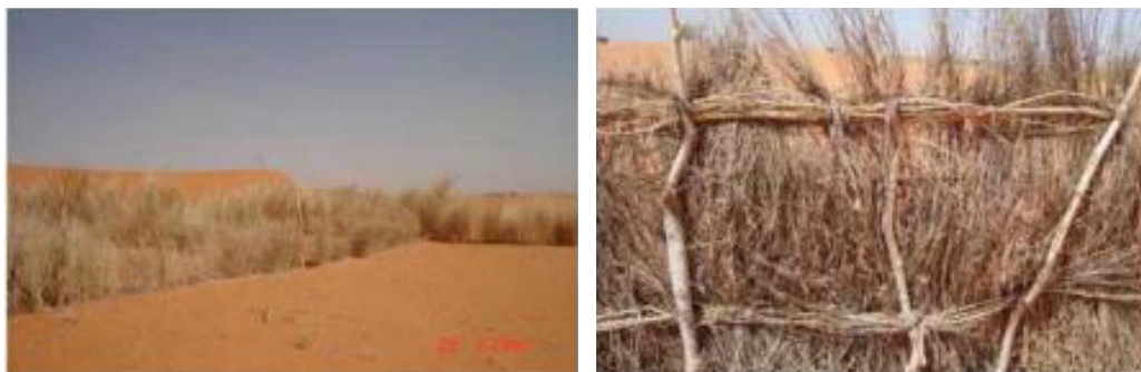
Mechanical fixation of sand dunes
