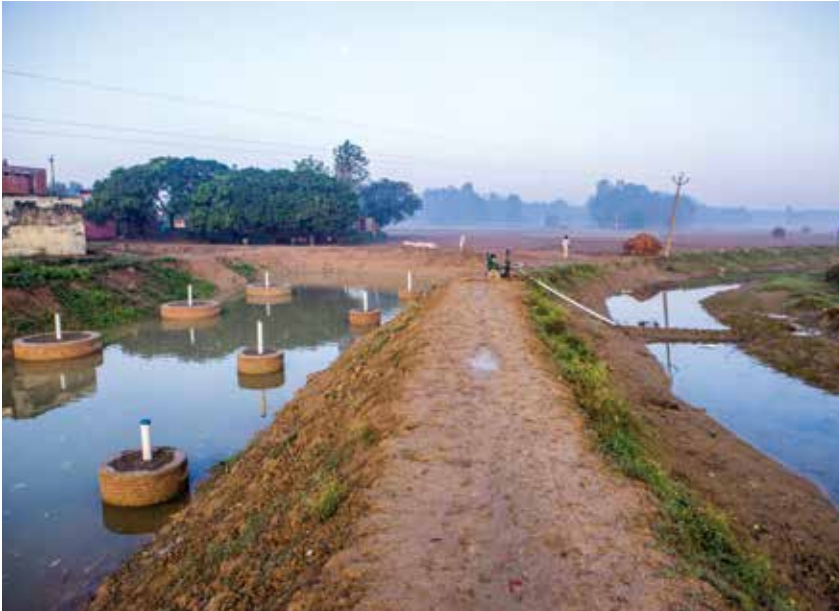
Pilot testing of aquifer recharge to reduce flood risk and make more water available for irrigation during dry spells in Uttar Pradesh, India.
