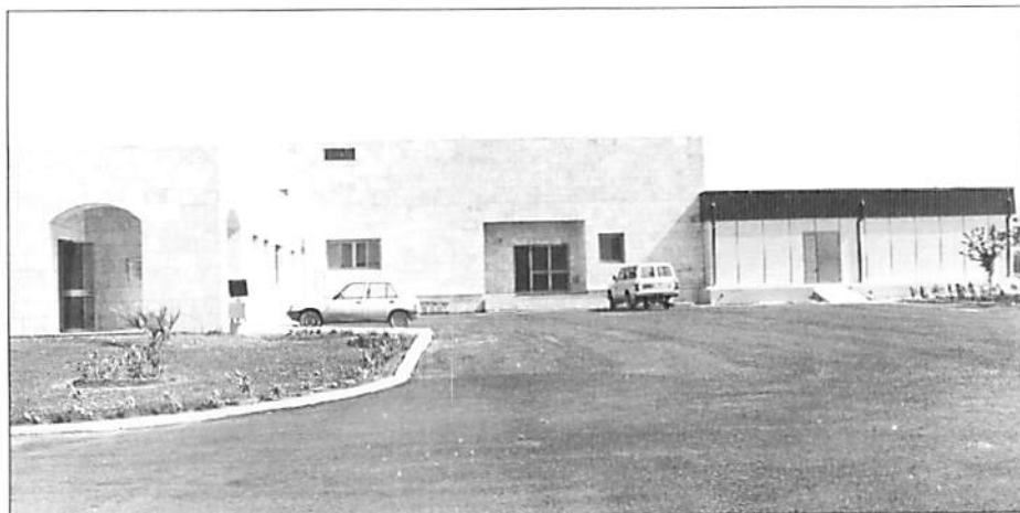
The new ICARDA Genetic Resources Unit at Tel Hadya, Syria (Photo courtesy of A.B. Damania)
