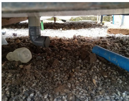
Plate 2.2. Bottom drainage in HS trough.
