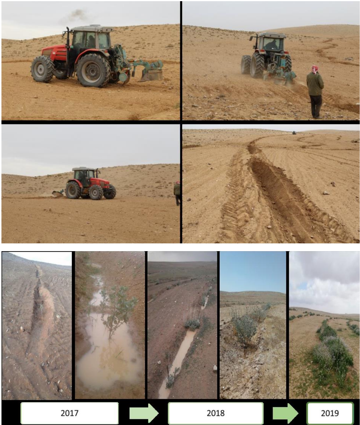
Photo 1: Vallerani Water Harvesting System. Photo Credit (Mira Haddad, ICARDA).
