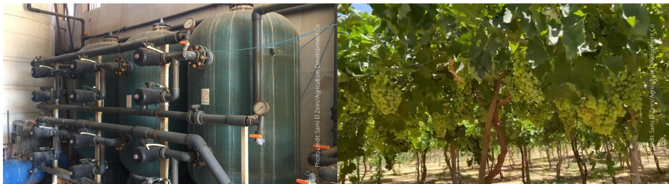
Plate 8. A desalination station for underground water (4500 ppm) (left), and grape trees irrigated with desalinated water (right) in the governorate of Giza.
