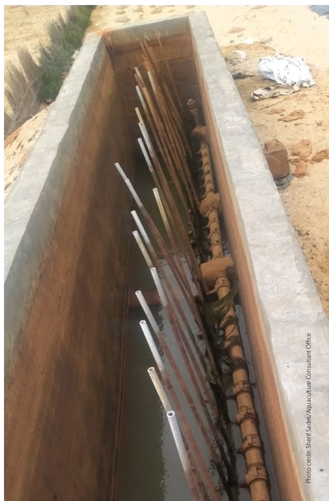
Plate 4. Iron oxidation tank using water-venture aeration to treat groundwater in Moghra.
