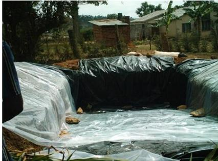
*Figure 5: A pit silo lined with polythene sheets*
