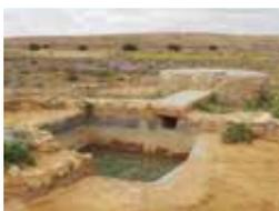
Natural or (hand) dug open reservoir to store water collected from elsewhere (Lasage and Verburg, 2015). The permeability of the pond can be reduced by using lining (concrete or plastic). Sizes vary from 30 m<sup>3</sup> (individual household use) to 20,000 m<sup>3</sup> (community use).
