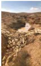
A check dam (also called gully plug) commonly constructed across a drainage ditch, swale, or channel having gentle slope to conserve stream flows and to conserve soil moisture. The harvested soil and organic matter act as a sand tank that quickly infiltrates stormwater flow, then slowly releases it to nearby plant roots.
