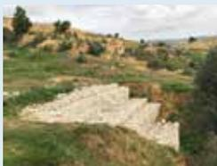
Stone gabion is constructed manually to treat deep ravine heads, to reduce the speed of water flow downslope, to capture soil flowing downslope, and to also reduce the effects of runoff on the soil.
