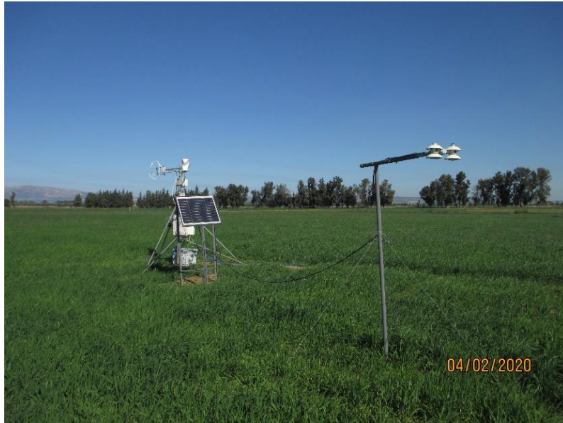
Fig. 11 - Location of the ET monitoring field site in Tunisia.
