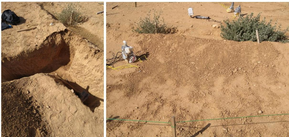
**Figure 10** Left: Picture of the cut used to install the Decagon 5TE sensors. Right: The Vallerani RWH structure after the cut was filled up.
