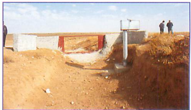
Low cost weirs may be installed on wadis to measure runoff rate from macro-catchments. This one is in Mouaqar, Jordan.
