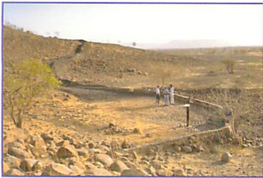
The hillside runoff system captures runoff water as it flows down the hill. (Photo by Prinz.)
