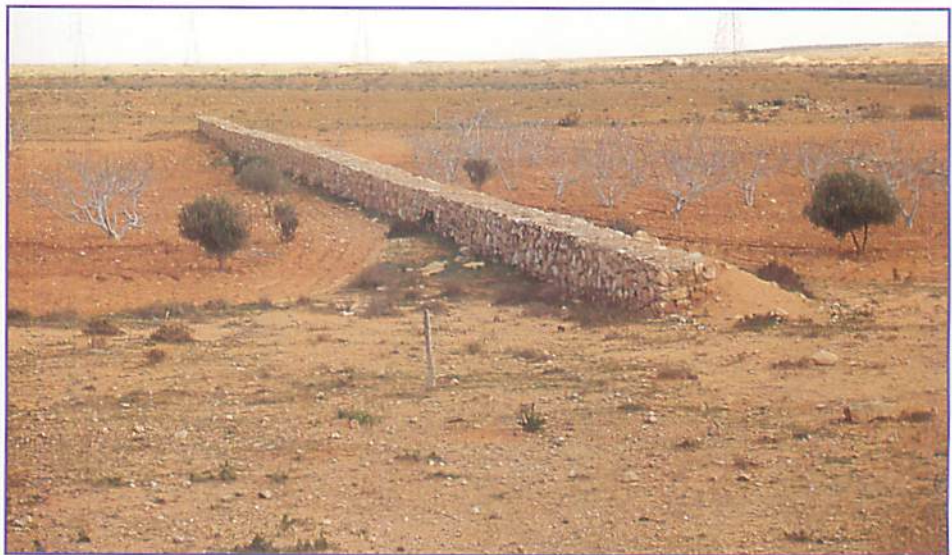
Stonewalls, if properly constructed across the wadi bed, can help to store and distribute runoff water evenly and to build up soil behind them.
