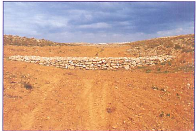
Stonewalls, if properly constructed across the wadi bed, can help to store and distribute runoff water evenly and to build up soil behind them.
