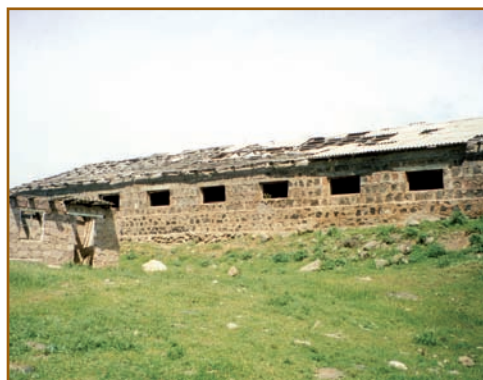
Production infrastructure dismantled
