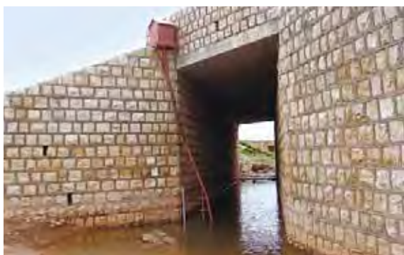
Figure 3.16. Downstream view of Charvarish Bridge with installed logger.
