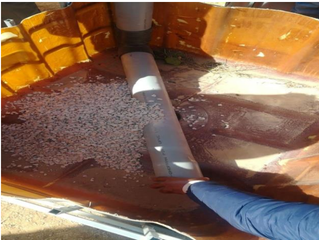
3- Add gravel on the pipe and covering the pipe to save and absorb water
