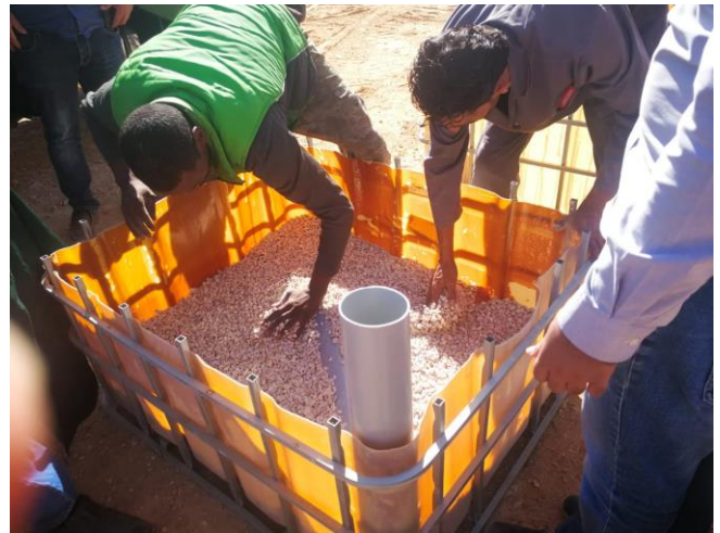
3- Add gravel on the pipe and covering the pipe to save and absorb water
