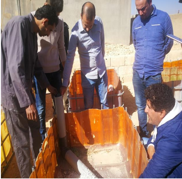
3- Add gravel on the pipe and covering the pipe to save and absorb water
